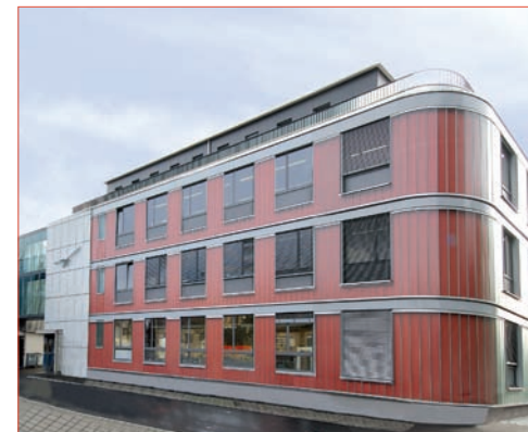
St. Gallerstrasse 116 (red corner)
