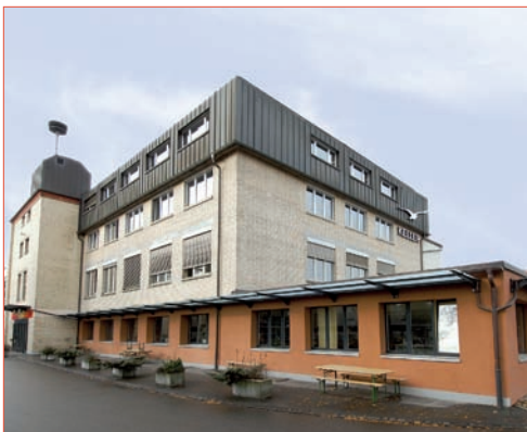
St. Gallerstrasse 119 (headquarters)
